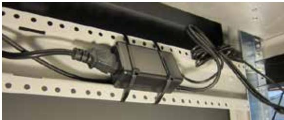
Figure 2 – Radio 12V DC Power Supply
