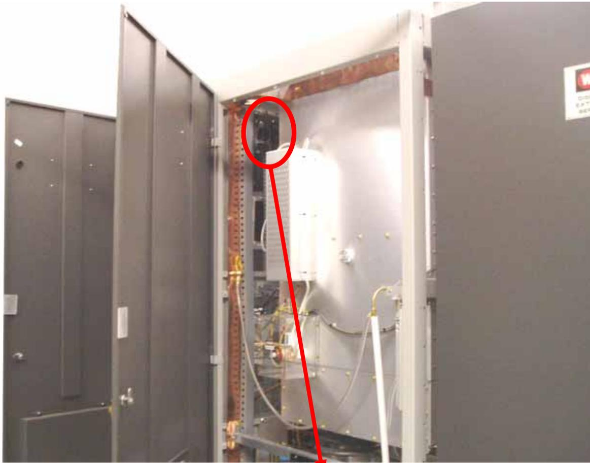
Mount the Attenuation Control PCB (919-0299) to the cabinet rail as shown using Qty (2) Standoffs (441-0101), Qty (4) #10 Split Locks (423-0002), and Qty (4) #10 Phillips Screws X .375 Long (420-0106).
