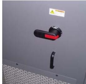
Figure 7 – 4MX Rear Panel AC Breaker
