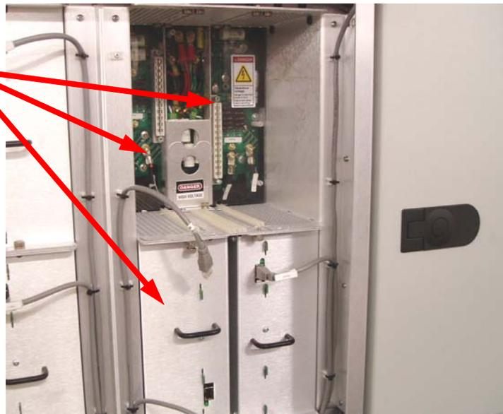
Figure 130 – Install PA Modules
