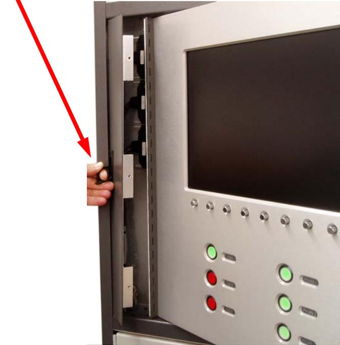
**Figure 23 – Multiplexer Access Panel Removal**
