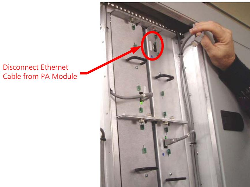
**Figure 102 – Disconnect Ethernet Cable**
