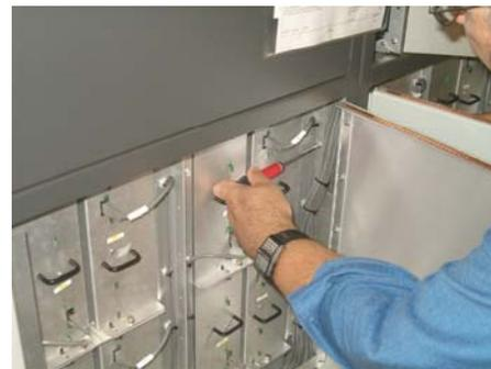
Figure 5 – Bolt 4MX 100 Main and Auxiliary Cabinets Together
