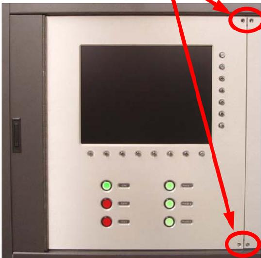
**Step 1b** – Use a No. 2 Phillips screwdriver and remove the (3) screws from the hinge area as shown
